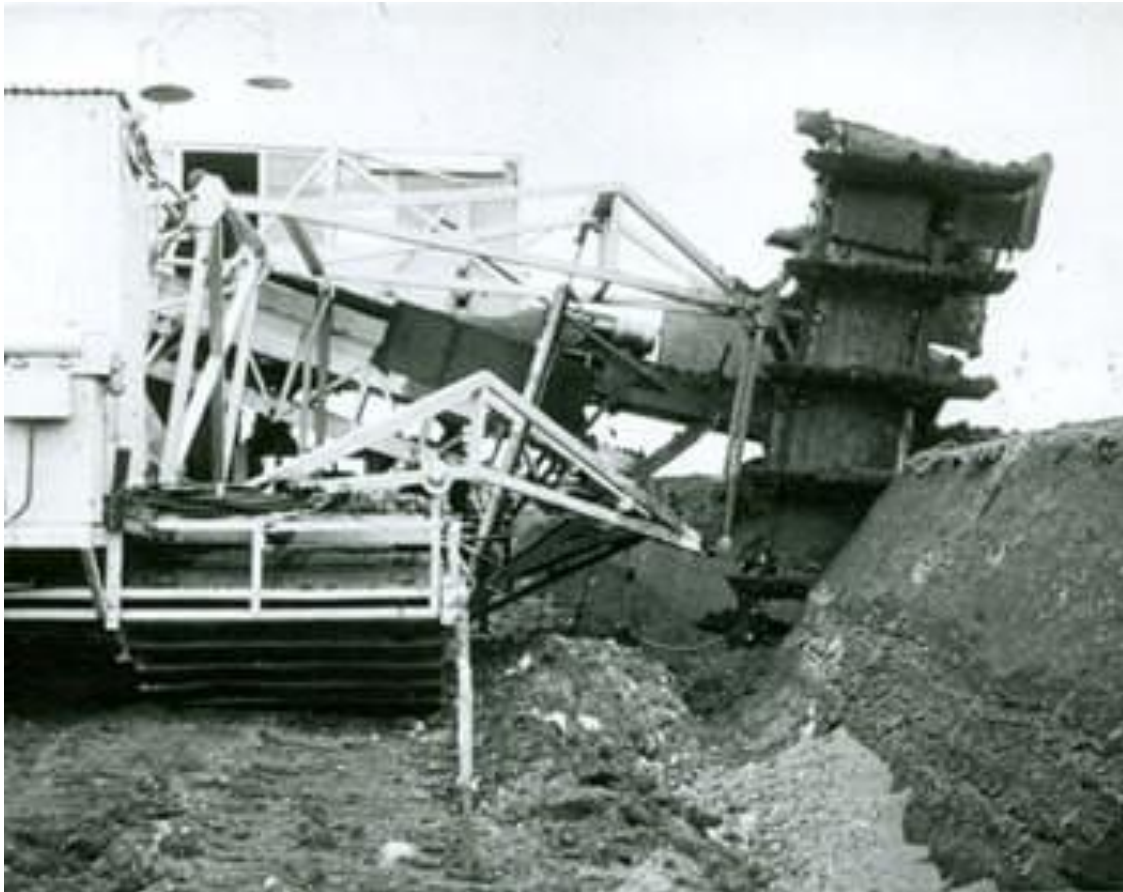
Plate 4-25 Cutaway Boom Attachment (source: Living History)
