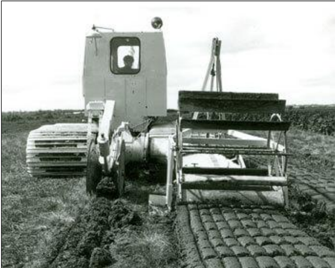
Plate 4-26 Chain Saw Excavator (source: Living History)
