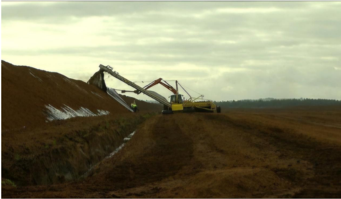
Plate 4-14 Polythene covering of stockpiles (source: BnM)
