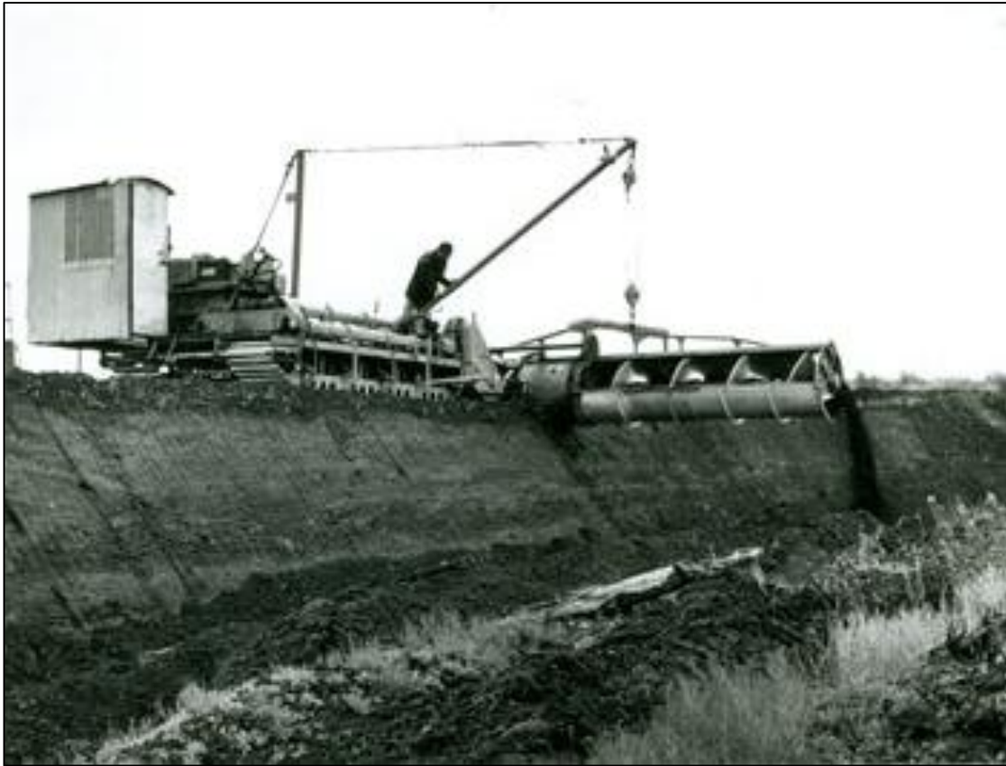
Plate 4-6 Stripping Machine (Source: Living History)
