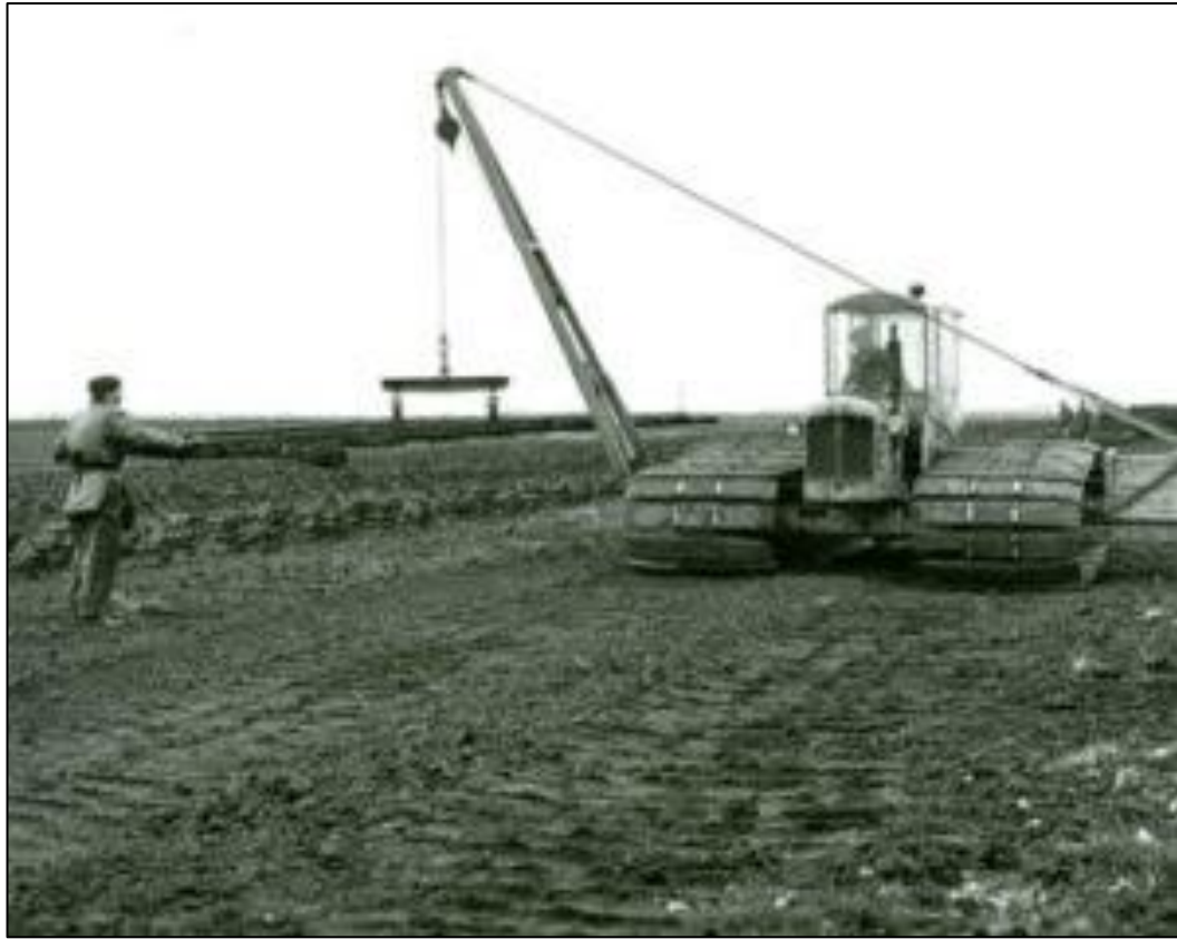
Plate 4-42 Rail Moving Attachment to lift and lay temporary track, along sod peat ricks and milled peat piles. (source: Living History)
