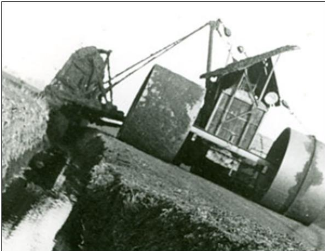
Plate 4-2 Drainage Machine Type – M.P. Field Slitter (Source: Living History)
